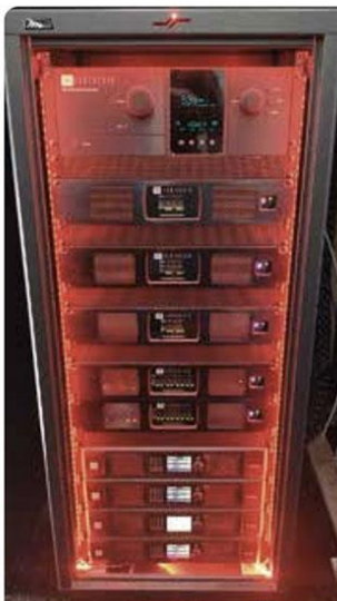
The system rack houses the SDP-75 processor and nine power amplifiers
